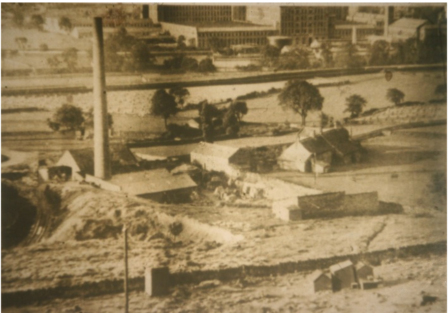
Baildon Green Brick Works, with Midgeley Farm on the right, Salts Mill in the far distance, and the curve of Green Road just visible on the left
